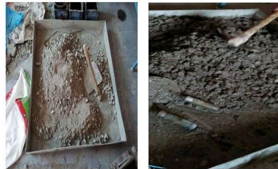
FIG: 4.1 BATCHING AND MIXING OF CONCRETE
